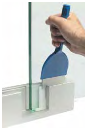
3. Hammer in the aluminium wedges
